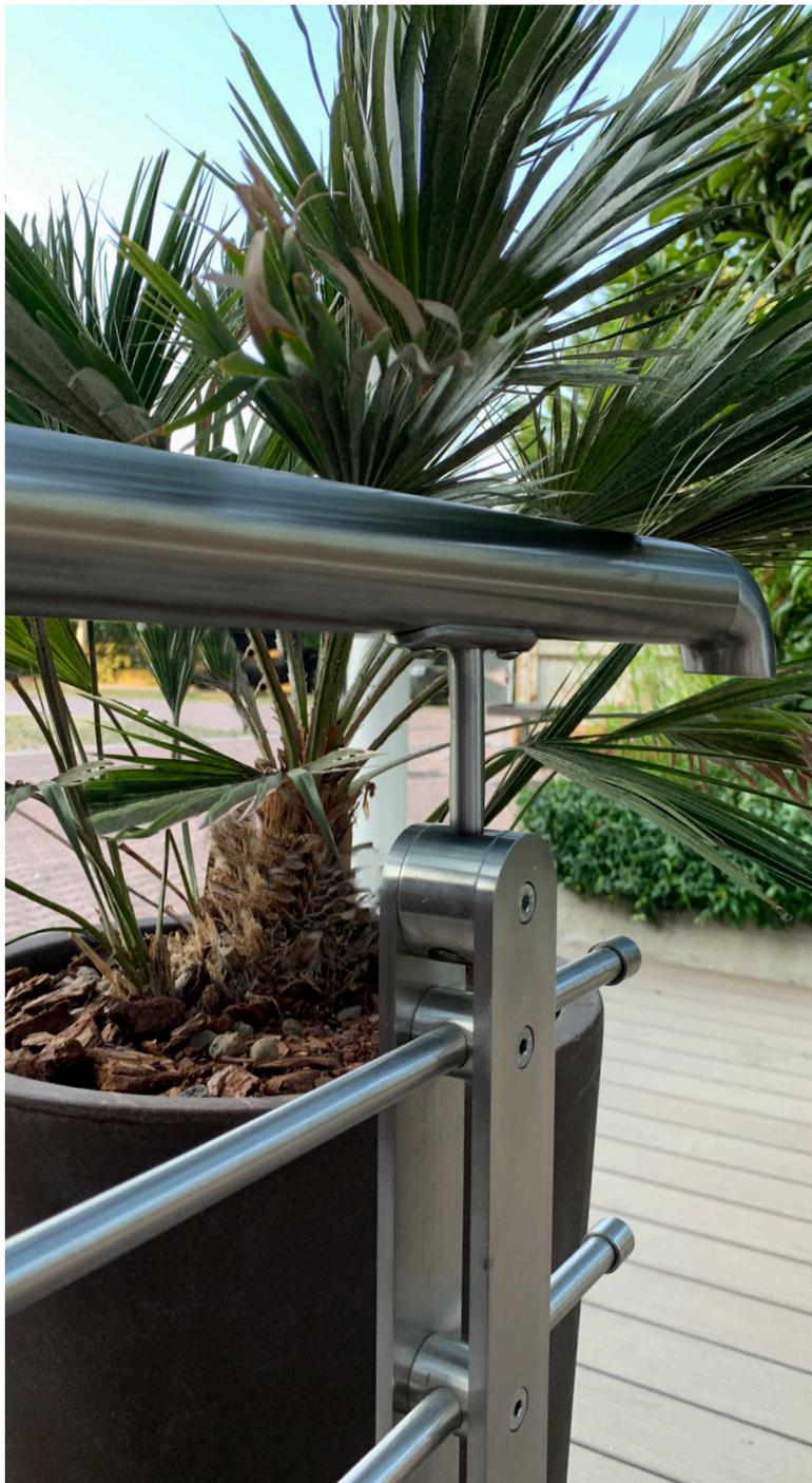
Two parallel structures joined together by supports that also act as round bar holders. Apparently complicated, instead absolutely simple.
